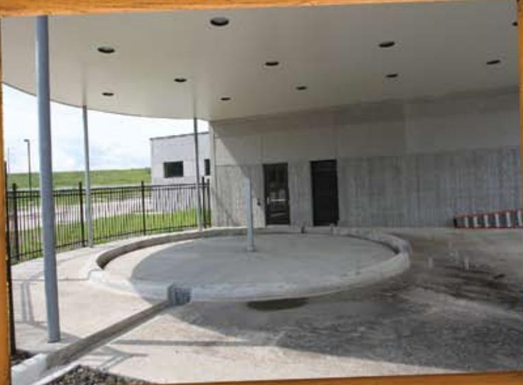
*This is the bovine unloading tub. Swing gates will be hung in the middle and the wall panels will be installed soon after.*
